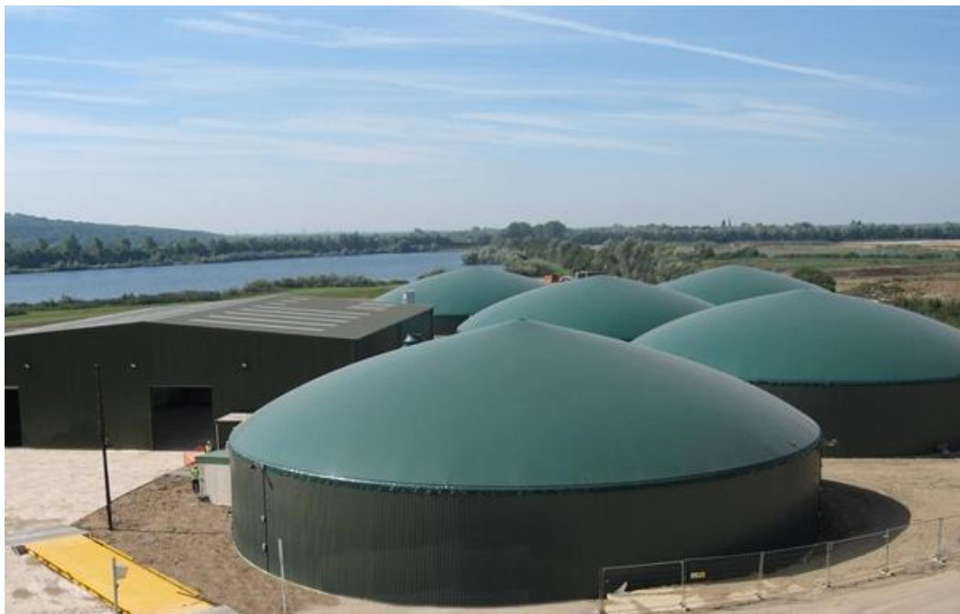
Figure 5.4: A Wet Anaerobic Digestion Plant
