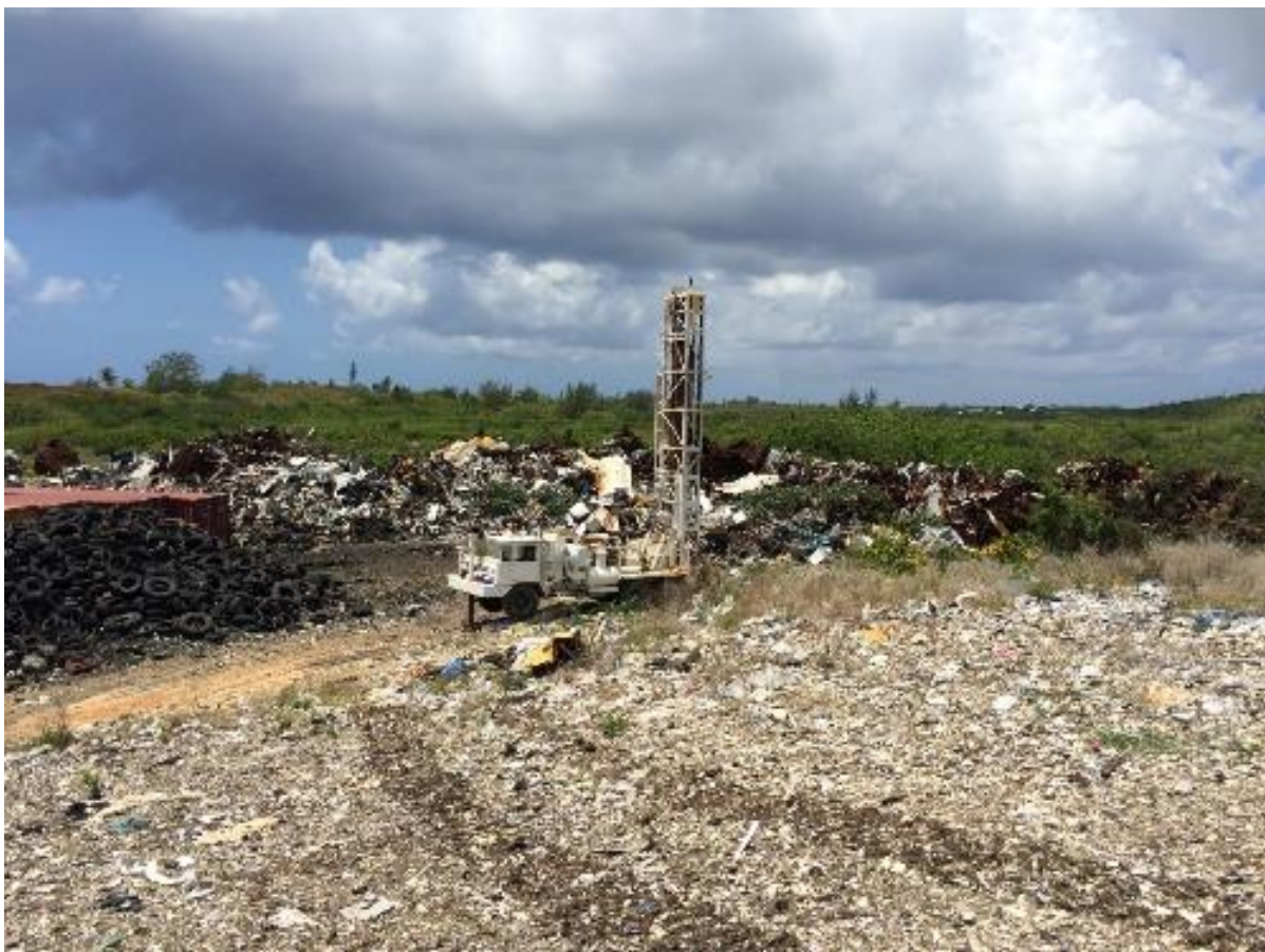
Figure 3.2: Borehole Installation on Cayman Brac
