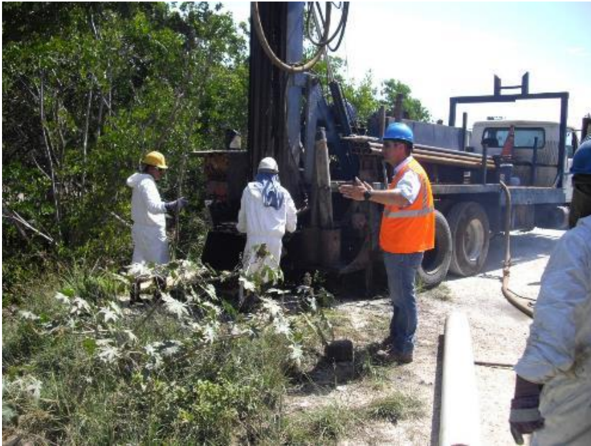
Figure 3.3: Borehole Installation at George Town landfill
