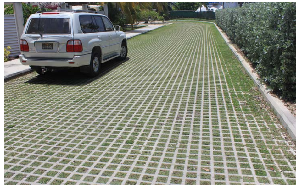
Figure 7.7: Porous paving surfaces can help to reduce surface runoff.
